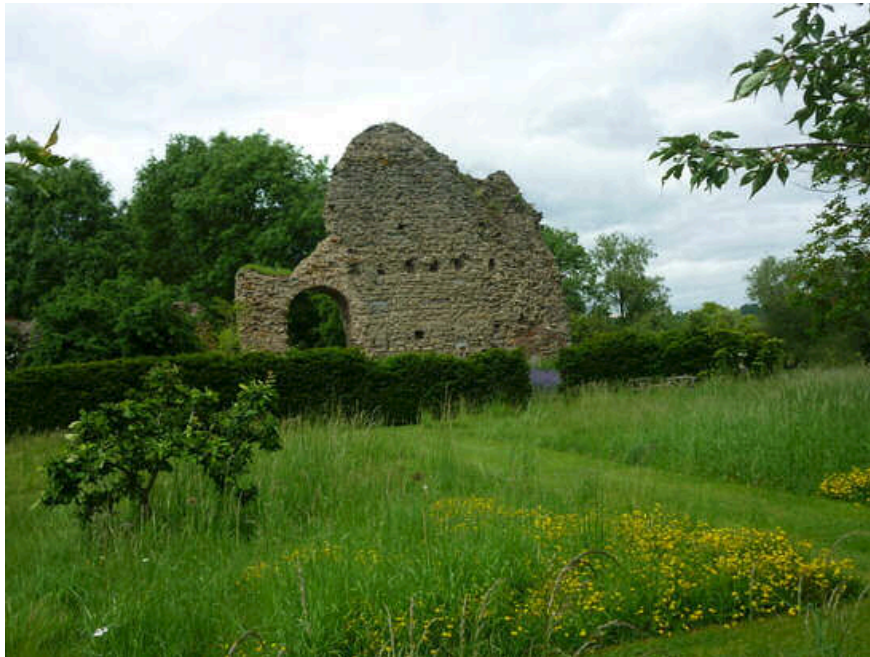
Part of the south transept survives to a good height
