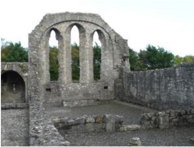
The church of St John the Baptist of the Crutched Friars at Newtown Trim
