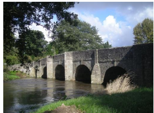
The 18th century bridge over the Teme at Leintwardine
