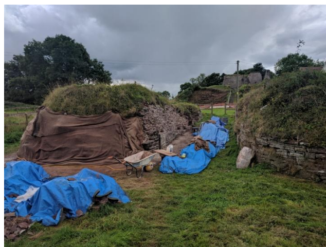
Work being done to stabilise the foundations of the gatehouse
