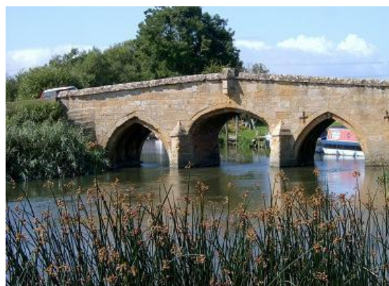
The original bridge at Radcot
