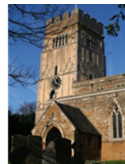
The tower of All Saints Church, Earls Barton displays limestone pilasters and long vertical quoins. Above the clock you'll spot a triangular-headed window.
