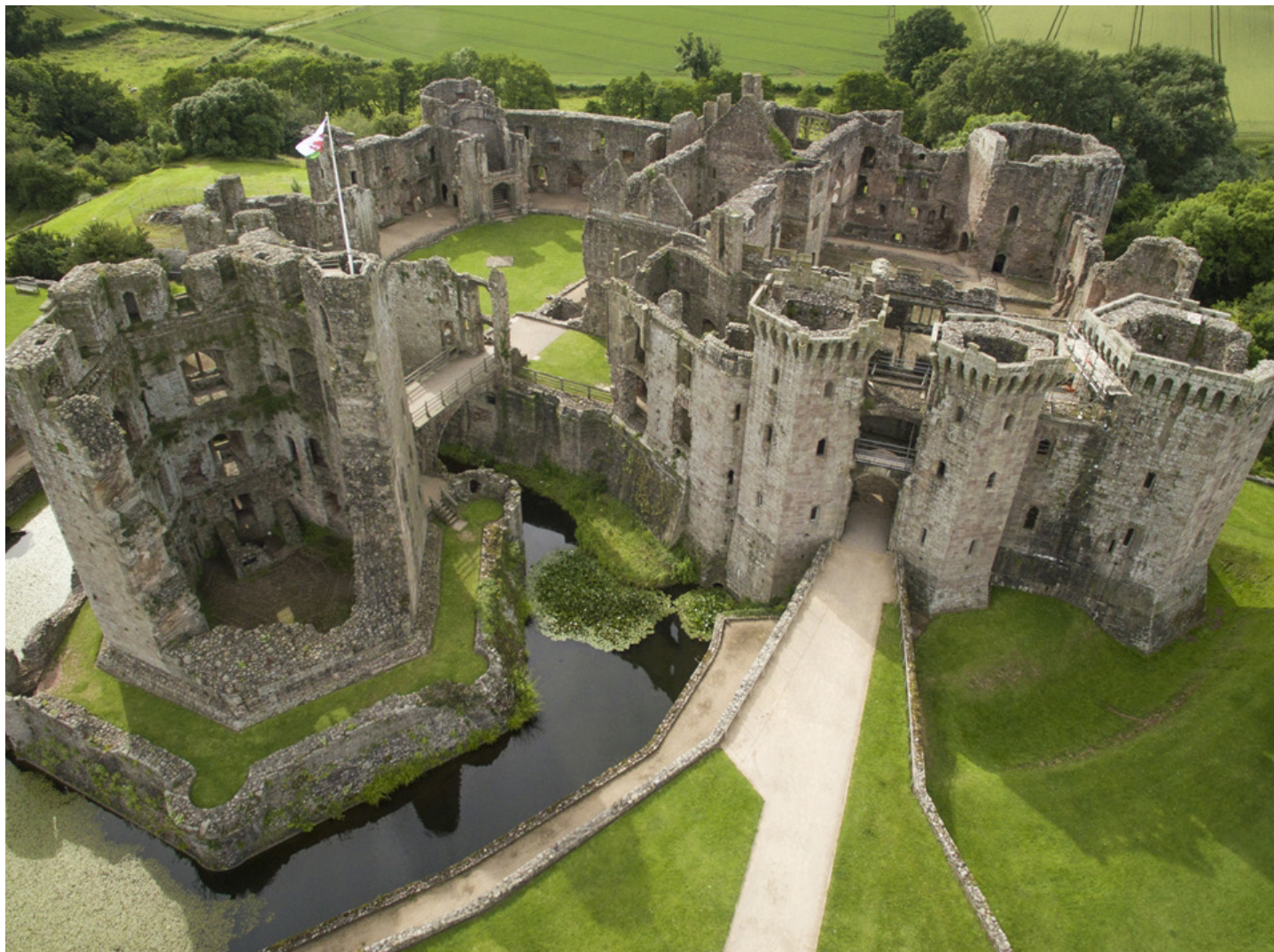
Raglan Castle, showing the gatehouse with its flared 'machicolations', one of the many additions commissioned by Lord William Herbert. ©Visit Monmouthshire.
