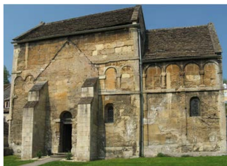
The blank arcade at St Laurence's Church, Bradford on Avon is characteristically simple.
