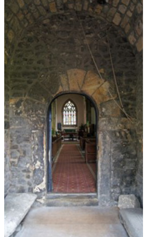
The porch under the west tower of St Peters in Monkwearmouth shows a vaulted roof of the simplest form.
