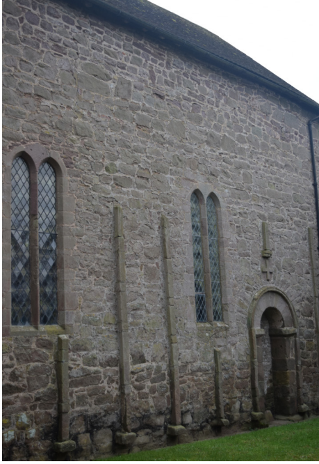
The north wall of St Peters, Stanton Lacy, showing decorative pilasters
